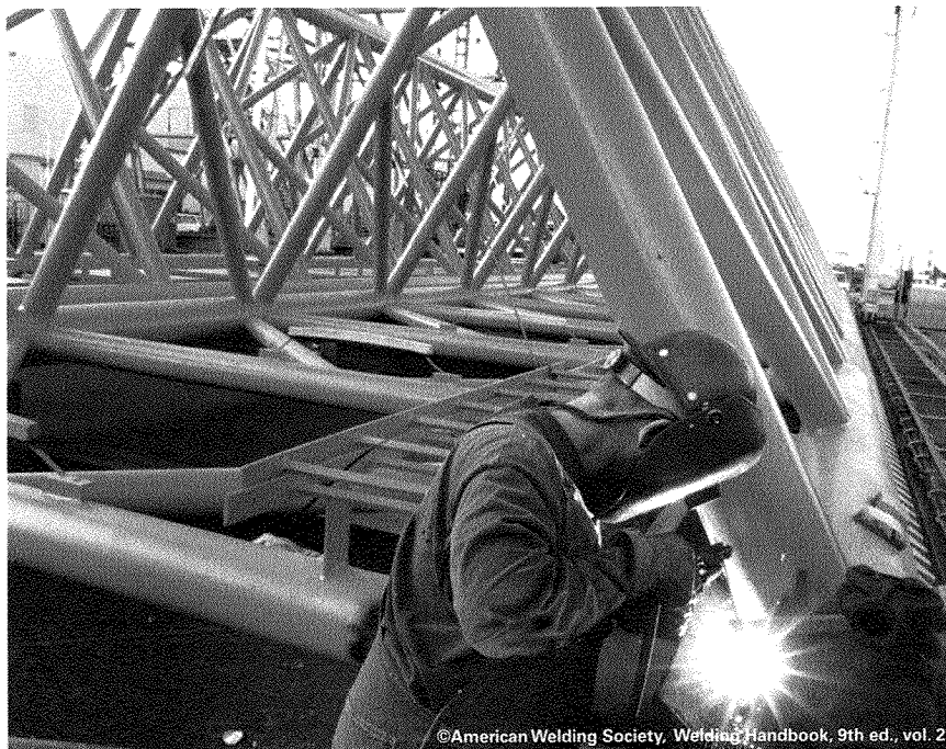
Shielded metal arc welding (or "stick welding")
