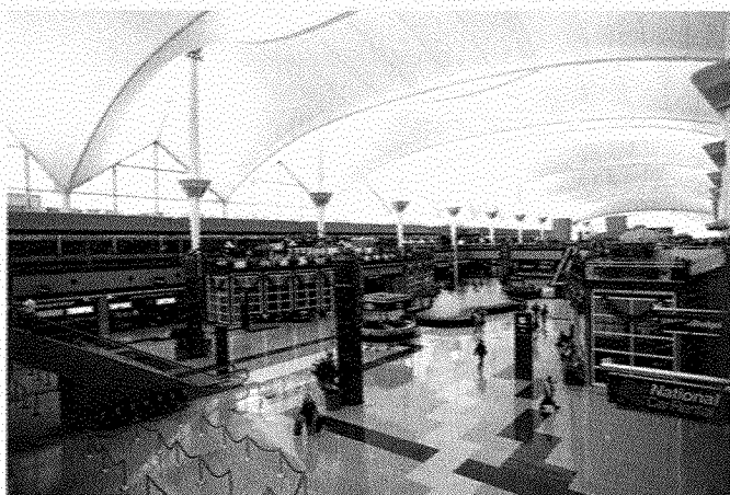
The fabric roof of the Denver International Airport lets natural light in during the day.
