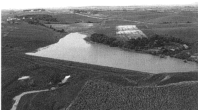
Watershed dams like this one help control runoff from streams and hold and store sediment.
