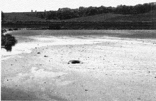
In large amounts, such as caused by accelerated erosion, sediment can be a pollutant and create costly problems. This small reservoir is rapidly becoming filled by sediment.
