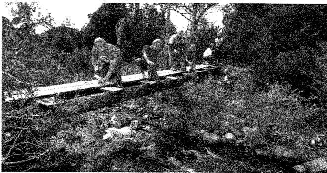
These Scouts repair a footbridge across a mountain stream. Conservation work became even more visible with the launching of Scouting’s Project SOAR (Save Our American Resources) in 1970.
