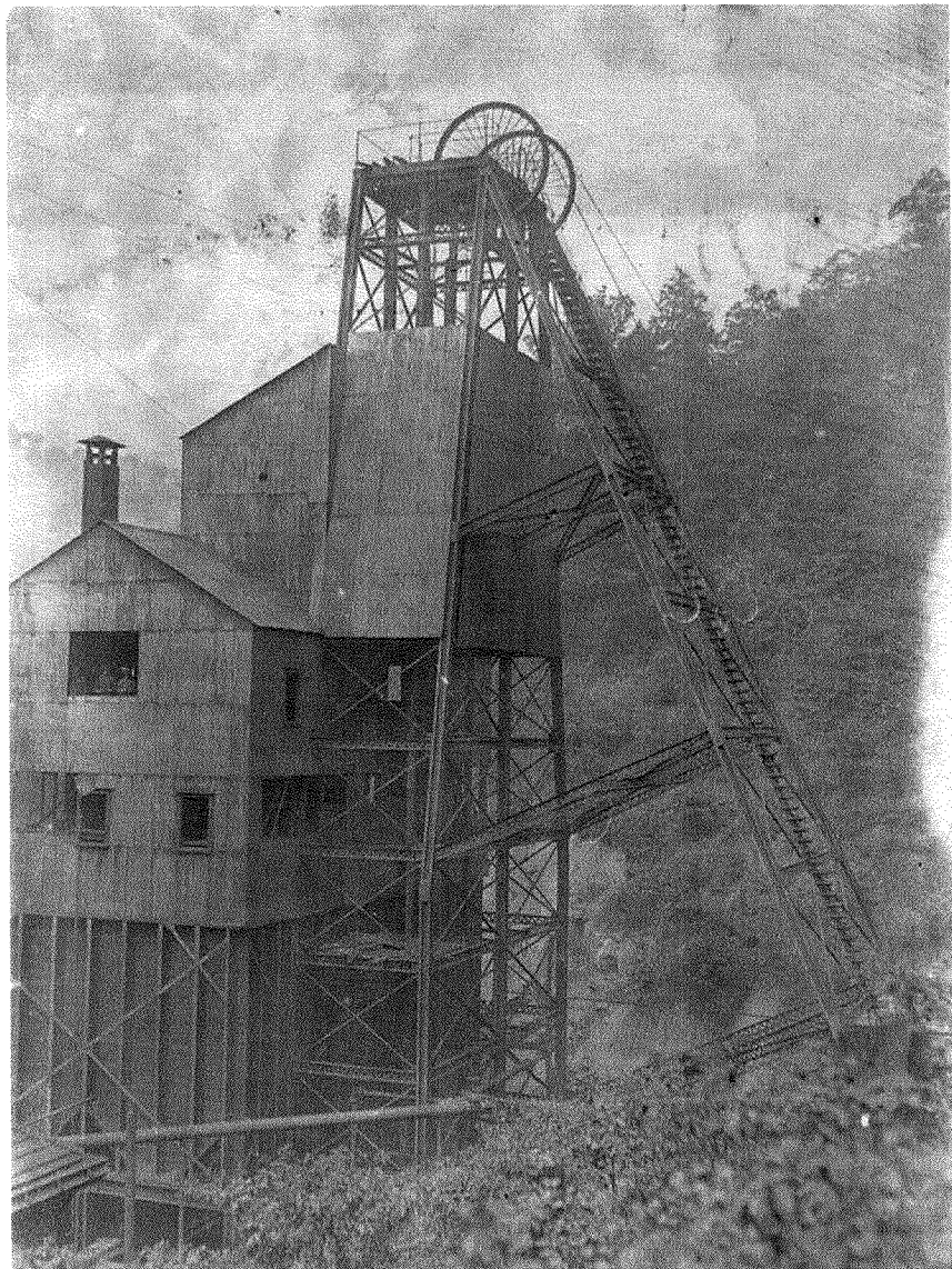
The smokeless coal formerly mined from the land of the BSA Summit fueled the steam shovels, steam drills, steam trains, and steamships that built the Panama Canal in 1904–1914. This photo shows a mine and tippie. Coal was lifted from the mine to the surface and prepared for shipping.
