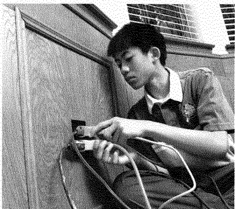
Too many cords are plugged into this outlet.
