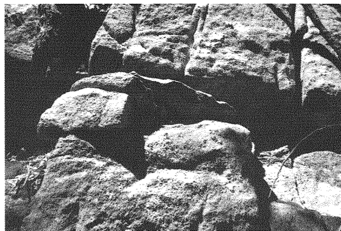
Crumbling and excessively fractured rock face
